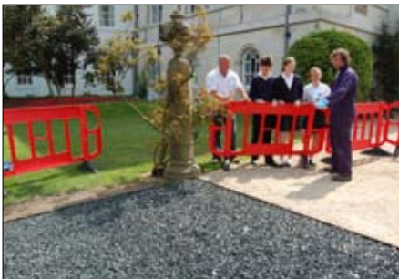
Pouring the easylay™ recycled tyre rubber mixture
