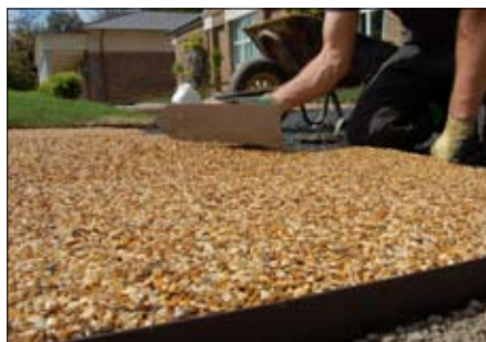
The easylay™ paving provides a full porous surface, which allow water to drain back to the water table
