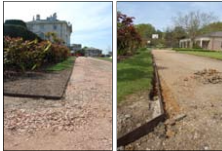
EverEdge was installed to create an edge to work up to. www.everedge.co.uk
